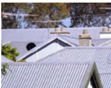
Galvanised iron sheeting
