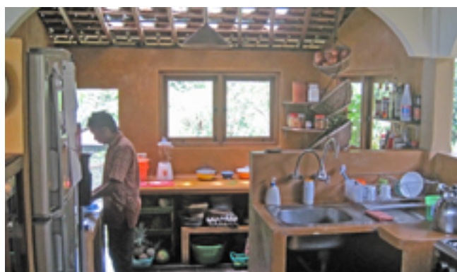
Ferro cement walls and countertops
