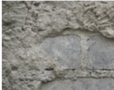
Local concrete w local clay slip
