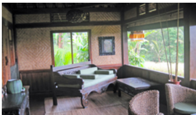
Woven bamboo walls & varnished floor
